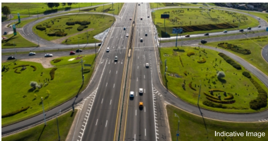
KGP/KMP Expressway Eastern/Western Peripheral Expressway
